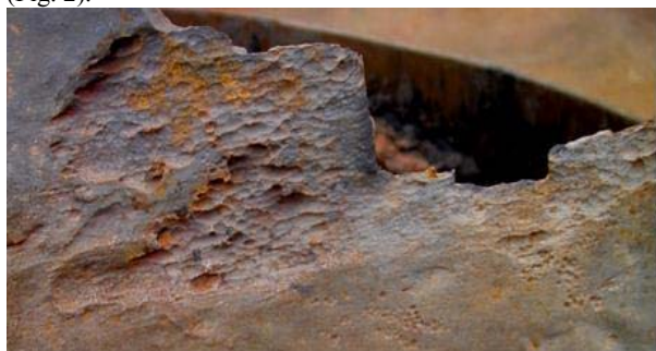
Fig. 1. Internal corrosion damages fragment pipeline pipes (steel grade 19Г)
